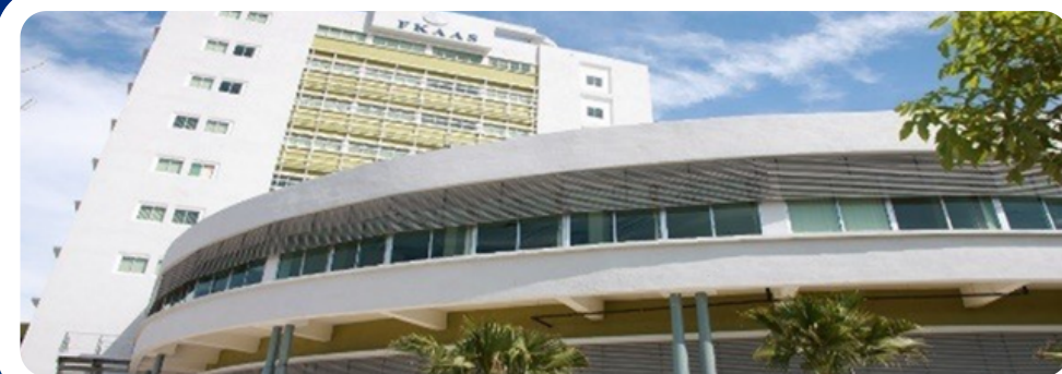
FACULTY OF CIVIL ENGINEERING & BUILT ENVIRONMENT
